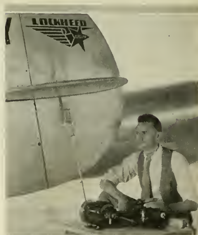
Determining stabilizer flutter characteristics of the Lockheed Electra
